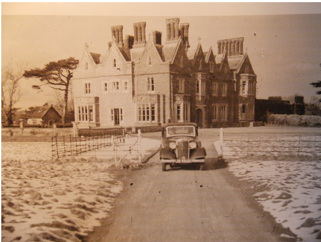
Figure 16: Arborfield Hall from the driveway
